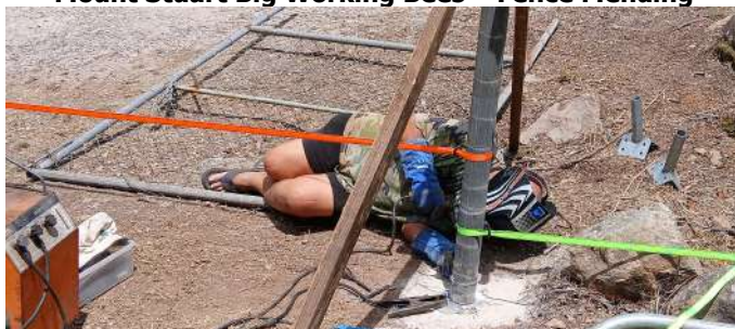
Snow/VK4ME does some horizontal welding on the gate post
