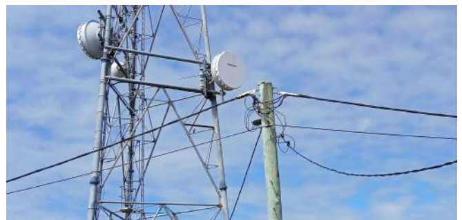
Ergon have replaced all the mains supply cabling around the site
