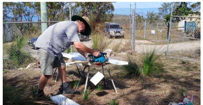
Phil/VK4HSV fabricates the new doorframes
