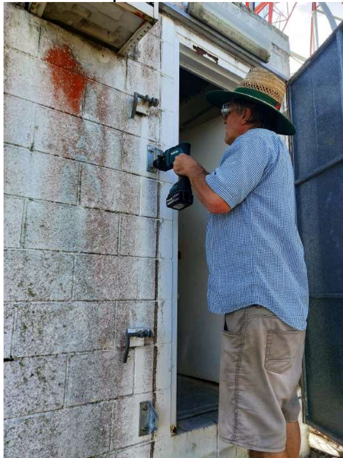
Phil/VK4HSV installing the locking plates for the Storm Door
