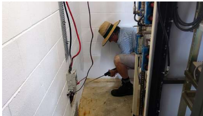
Phil/VK4HSV improving the draining holes in the hut
